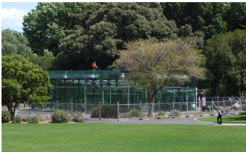
Figure 5 Construction Worker Cleaning Glass Roof – Viridian 'Activ' Coating will reduce the frequency by which this is required (photo Jeremy Prentice, DEH)
