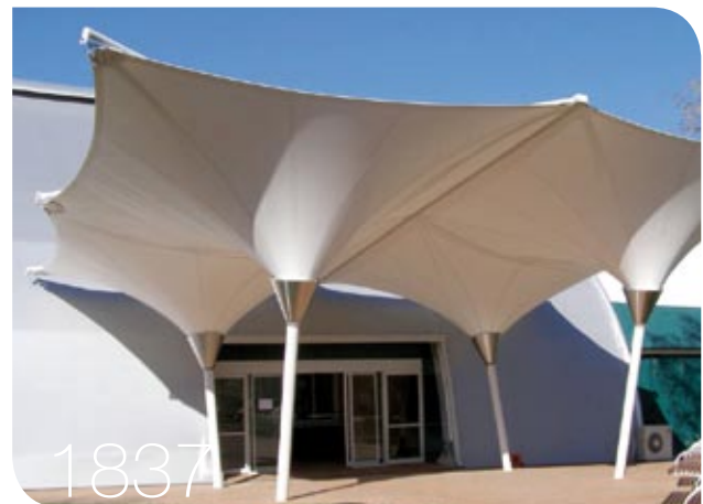
Mpowerdome Entry Structure
