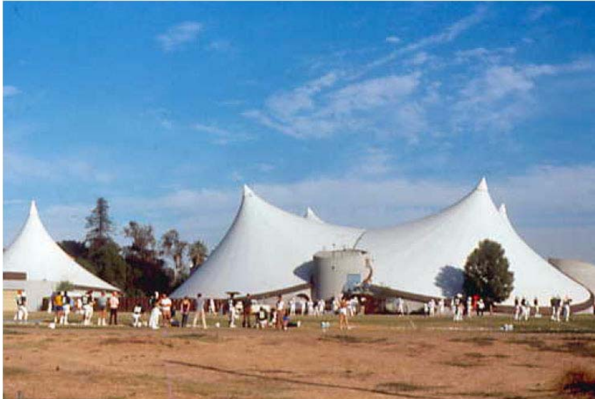
Figure 8 – University of La Verne Sports Science and Athletic Pavilion (California) Erected 1972, photo taken 1985
