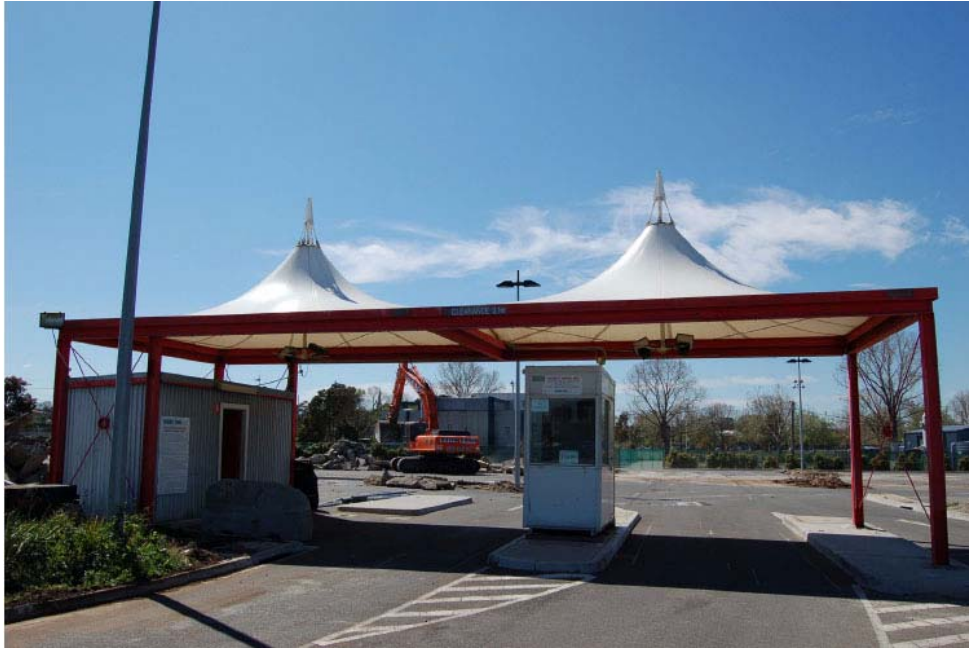
Figure 5 – twin conic in pvc-coated polyester with PVDF, erected 1990, photo October 2007
