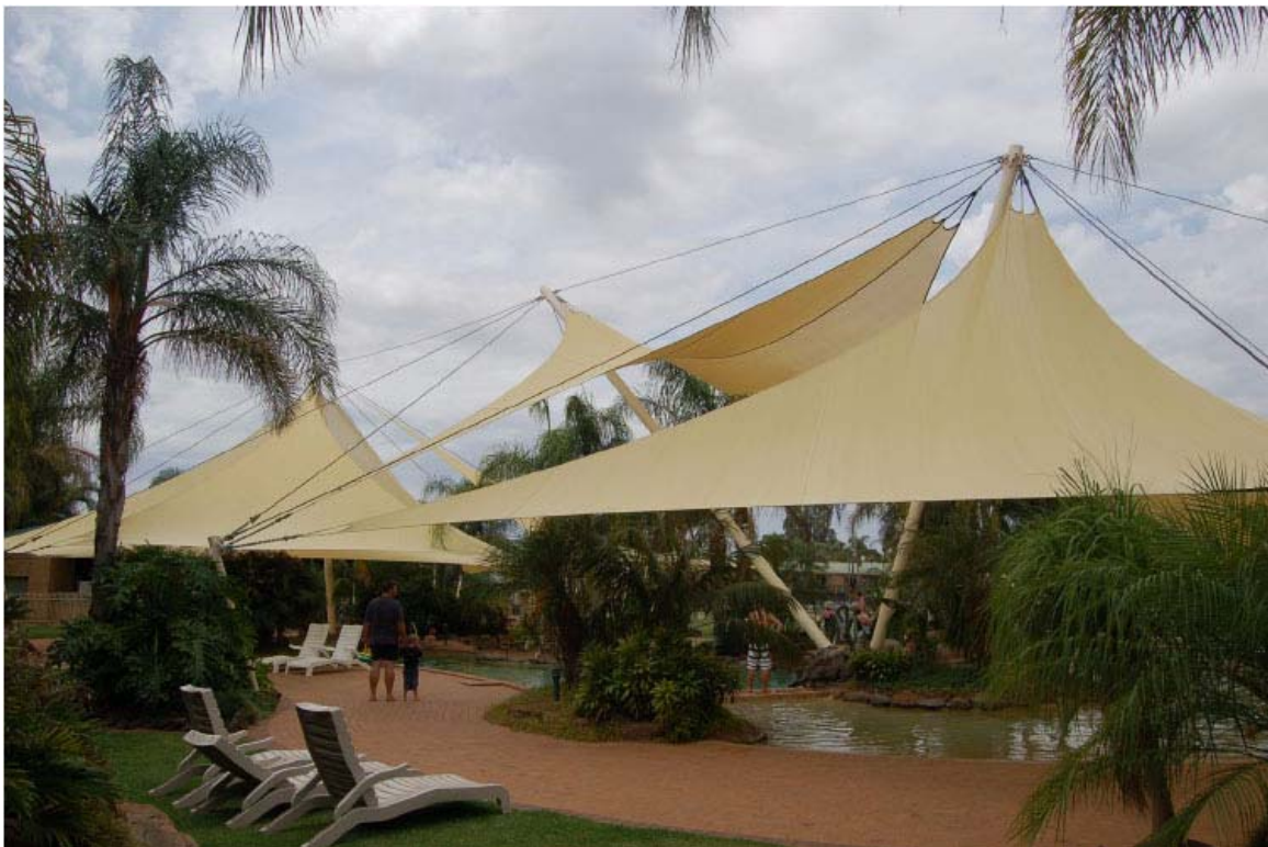
Figure 2 – Shadecloth canopies at resort in Northern Victoria Installed 1997, replaced 2006
