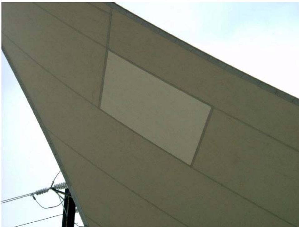
Figure 4 – repair of tear in PVC-coated Polyester membrane, installed 1996, repaired 2006
