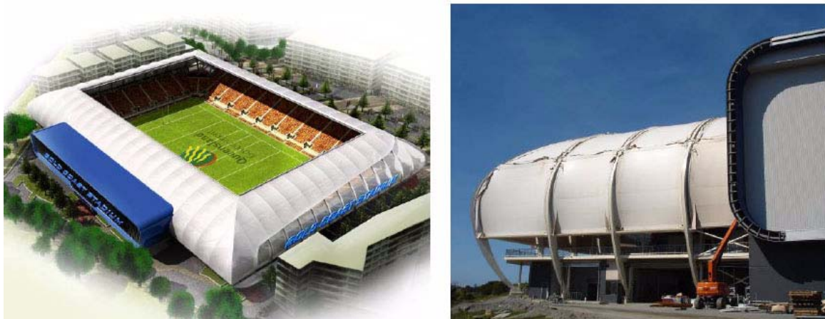
Figure 7. Presentation image showing west stand accommodation and September construction shot.
