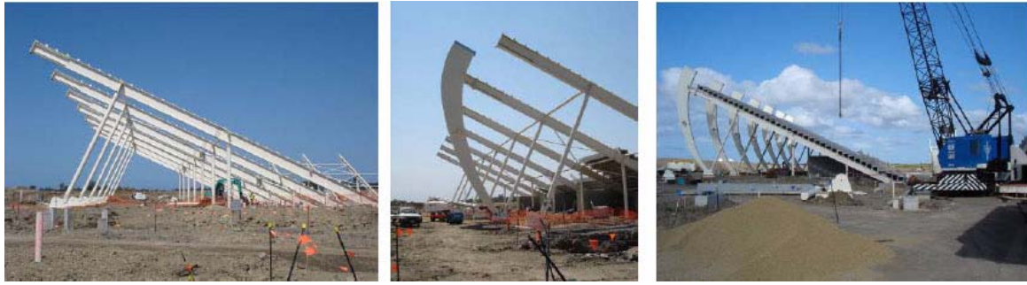
Figure 4. Images showing the sequential construction of the North stand.
