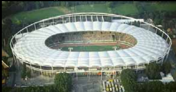
Gottlieb Daimler Stadium, Stuttgart A 70m clear span fabric roof with a minimal weight of 36kg/m 2 ACS4
