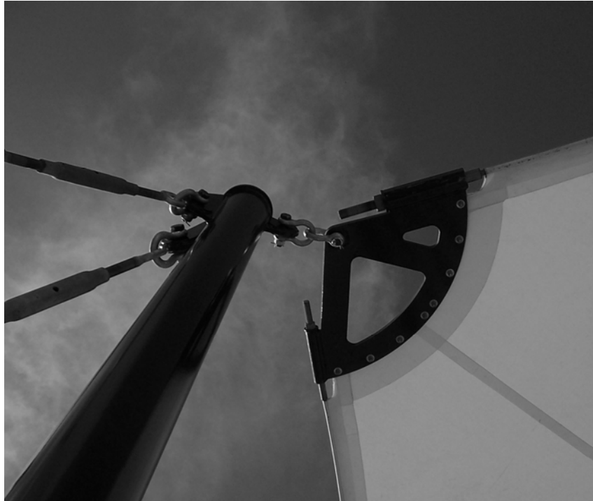
Image 8 – Typical Membrane Plate detail with galvanized fittings
