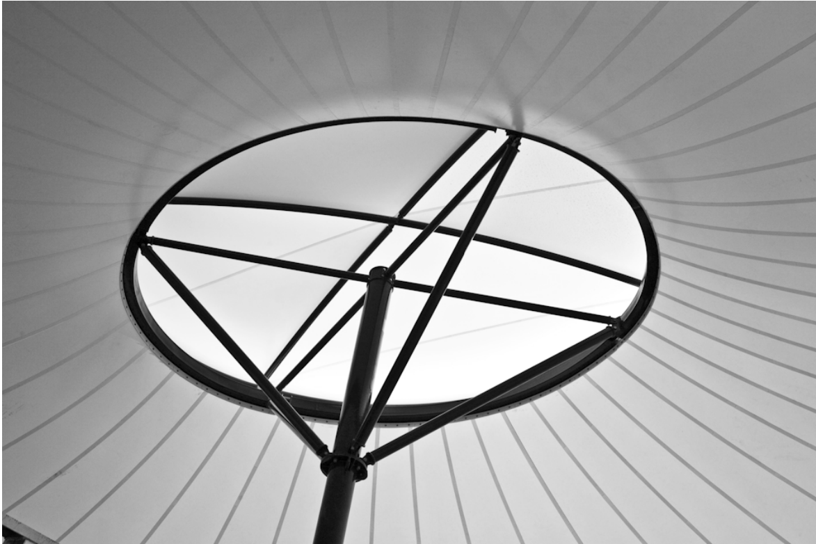
Image 7 – Contrast of High Translucency Cap Fabric with Main Fabric body
