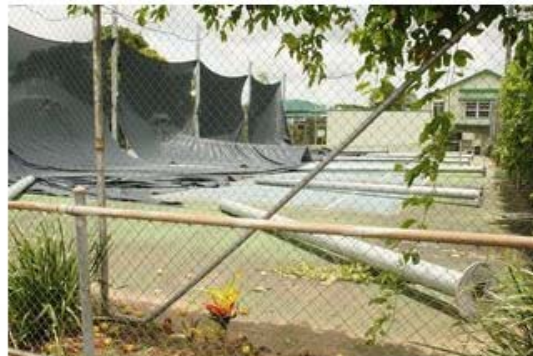
Safety concerns: Parents are worried shoddy workmanship may be to blame for the collapse of a shade cloth at Mena Creek State School.
