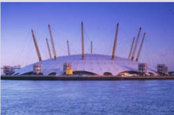
Millennium Dome – now the O 2 300 m diameter Built to provide an environmental enclosure for the Millennium Exhibition.
