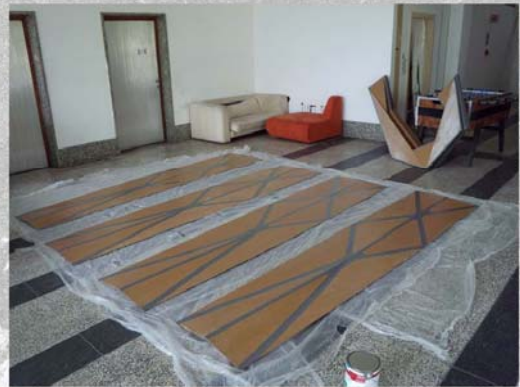
waterproofing of segments
