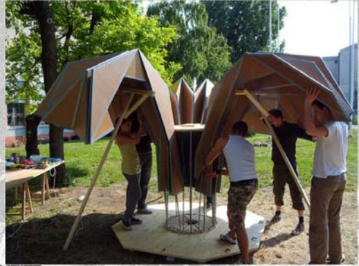
lifting umbrella onto assembly rig
