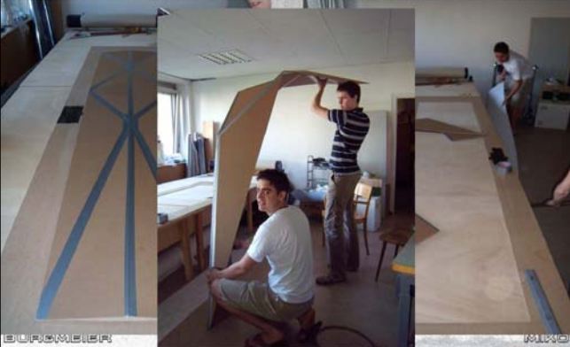
prototype construction: joining elements into segments
