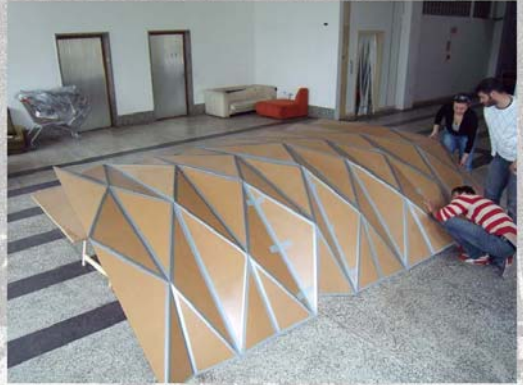
joining waterproofed segments
