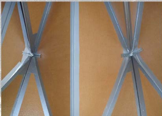
detail of taped joints and bolt connections to assembly rig
