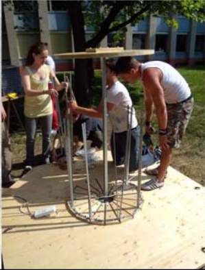
fixing anchoring straps for trunk to the assembly rig
