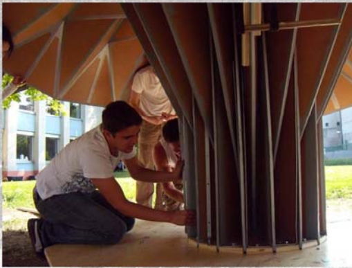
fixing anchor straps to trunk
