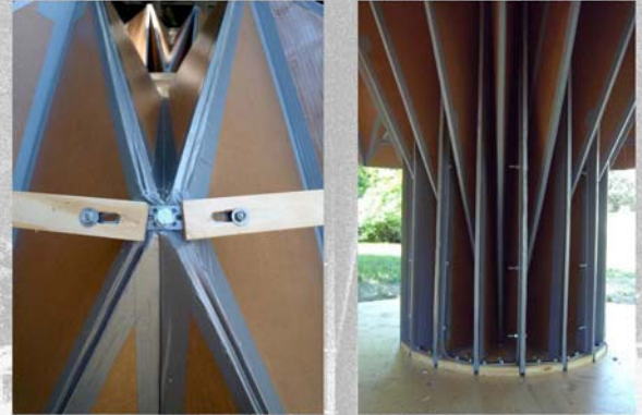
details of external bracing struts and trunk
