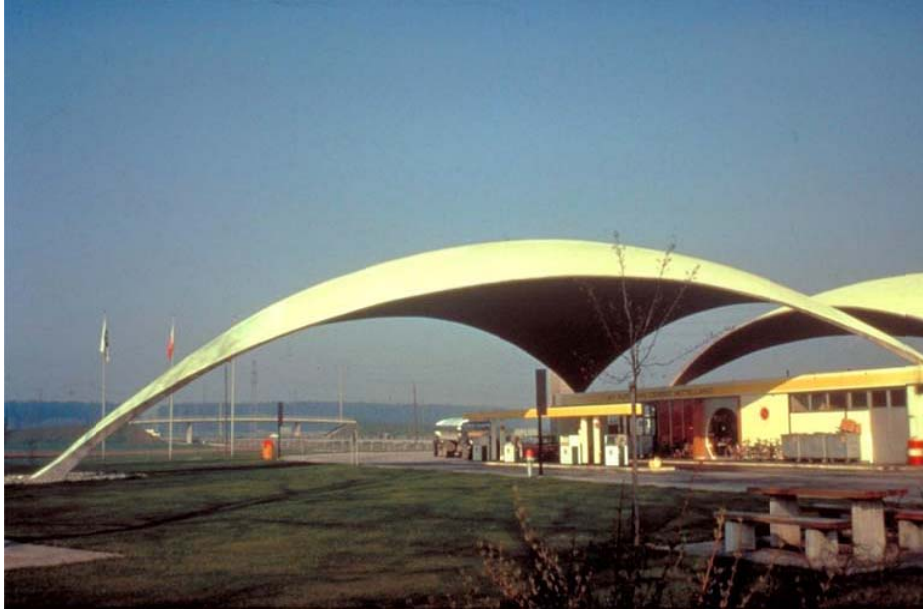
Fig. 4 Heinz Isler, Petrol Station in Deitingen, Switzerland, 1968
