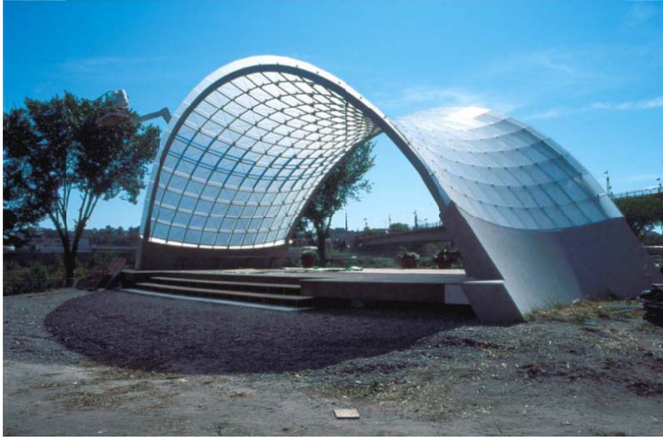
Fig. 11 Glass Hyper Roof with plane quadrangular Glass Panels, Schubert Club Band, Minneapolis, USA, 2001
