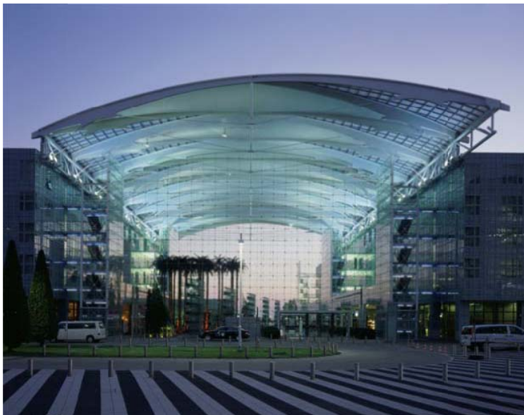
Fig. 7 The First Cable-Net Glass Façade, Hotel Kempinski, Munich, 1993
