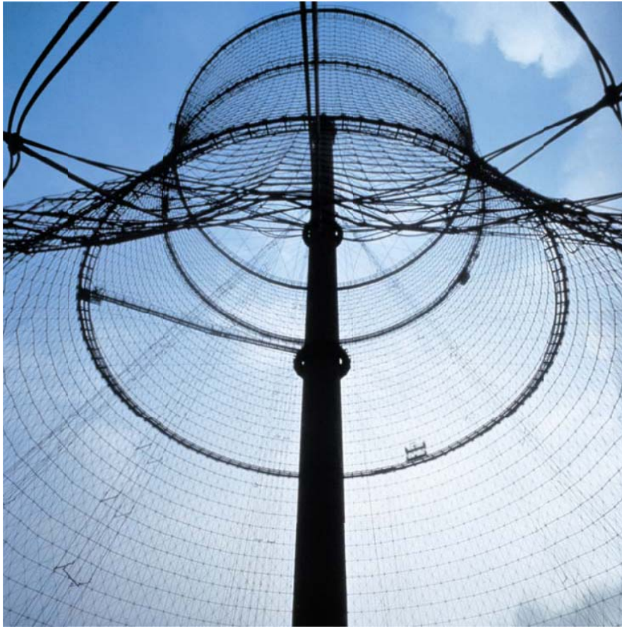
Fig. 8 Cable-net Cooling tower during construction, Schmehausen, Germany, 1974
