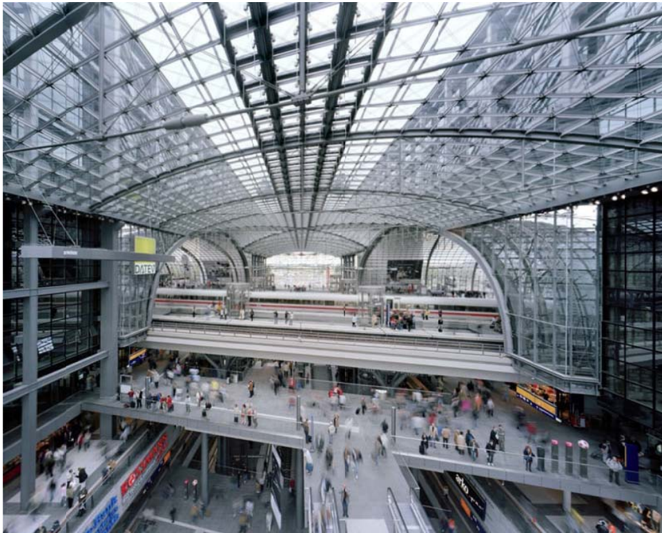
Fig. 12 Glass Grid Shells with plane quadrangular Glass Panels, Berlin, Main Station, 2006
