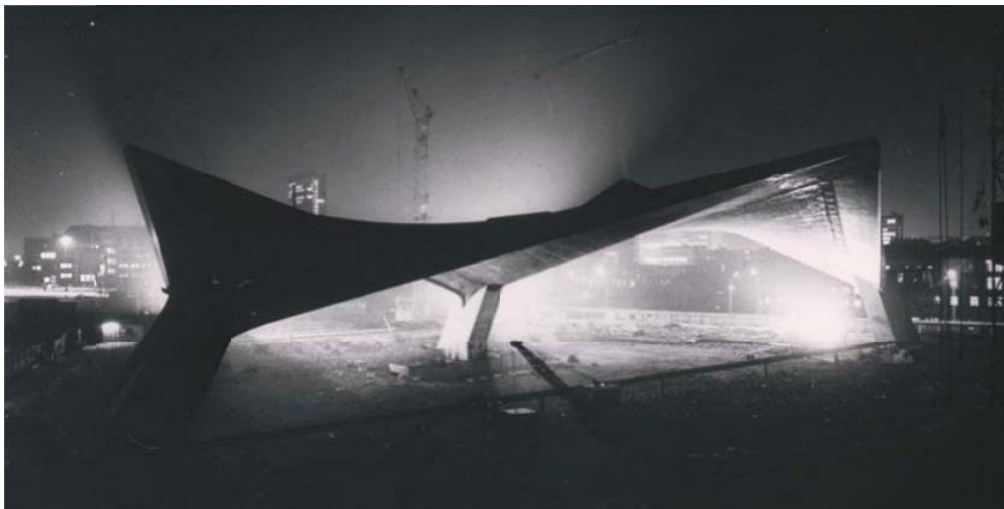
Fig. 3 Jörg Schlaich, Swimming Pool at Sechslingspforte, Hamburg, Germany, 1967
