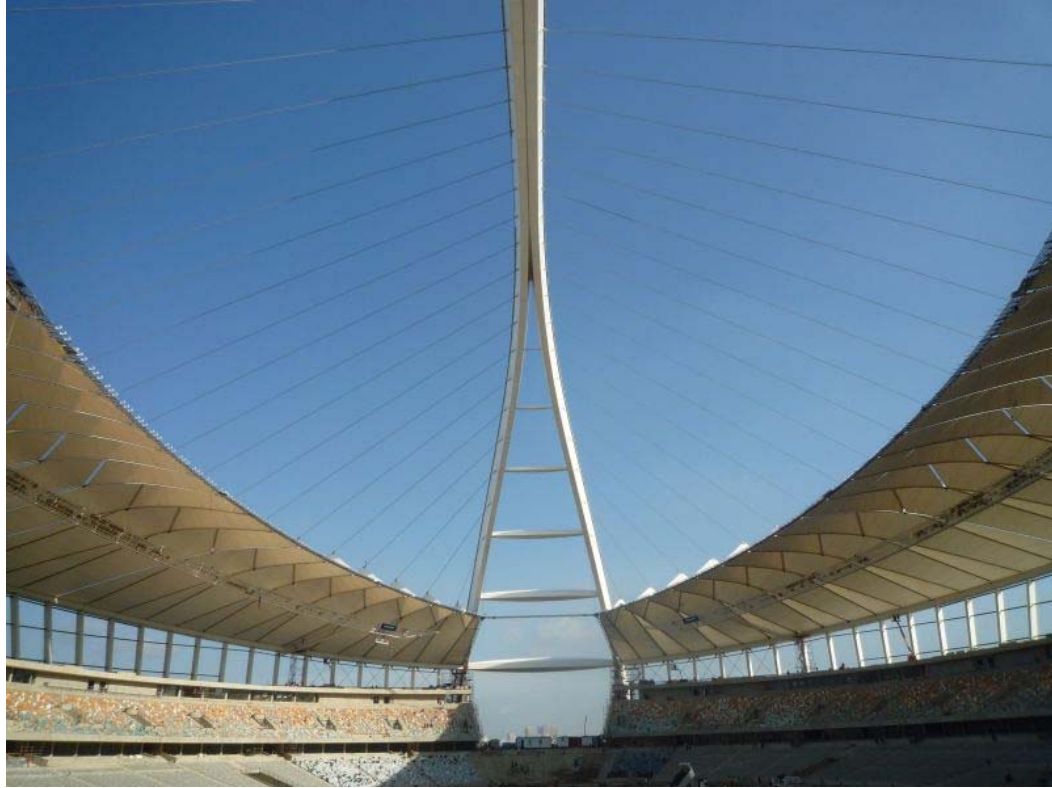
picture 16: Membrane panels in place
