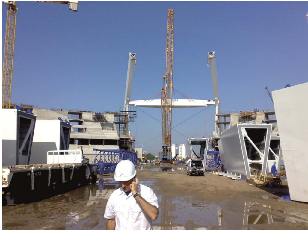
picture 7: Rung 1 has been installed
