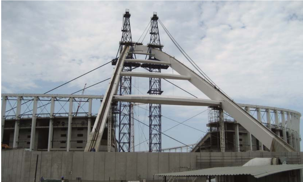
picture 9: Temporary towers with bracings and suspension
