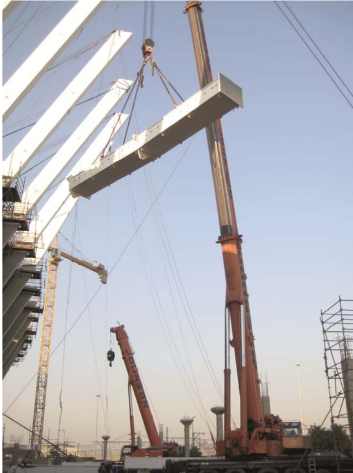
picture 13: Lifting a compression ring element
