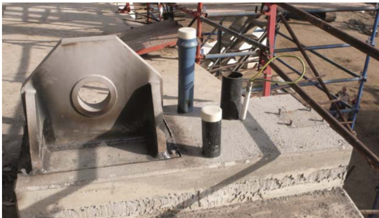
picture 12: Weld on lug for a column
