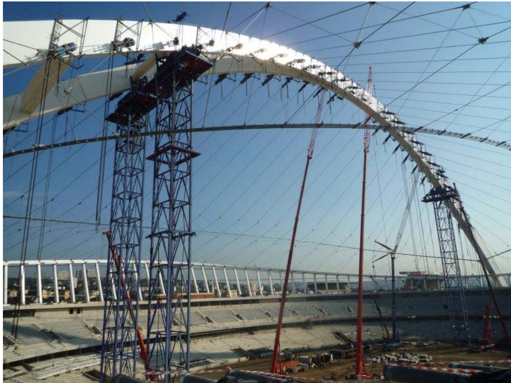
picture 15: Hydraulic jacks have climbed to the arch
