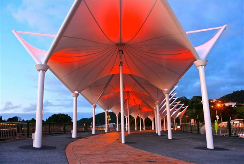
John Street Bridge
