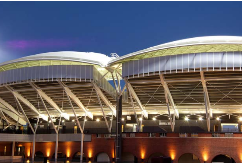
LSAA 2011 DESIGN AWARDS Adelaide Oval Western Grandstand Redevelopment
