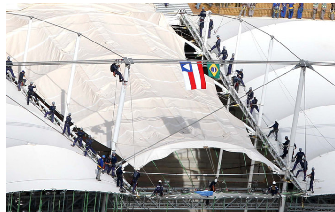
Last panel installation
