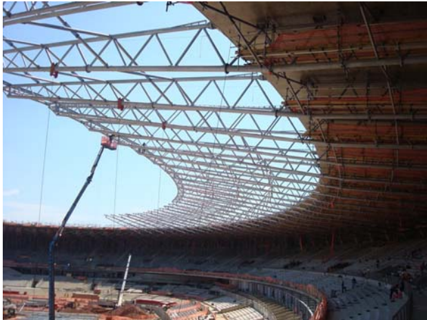
Add and level the cantilever section
