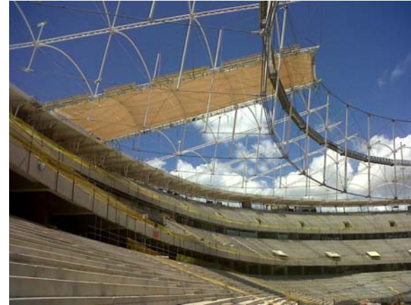
First panel installation
