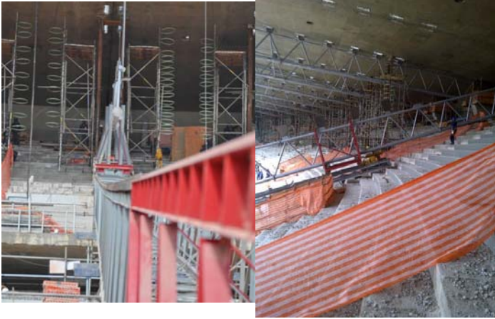
Lift the truss section into place
