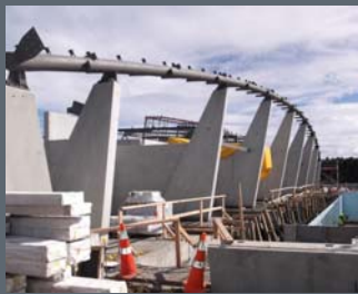
Precast Cantilever Column with Curve CHS
