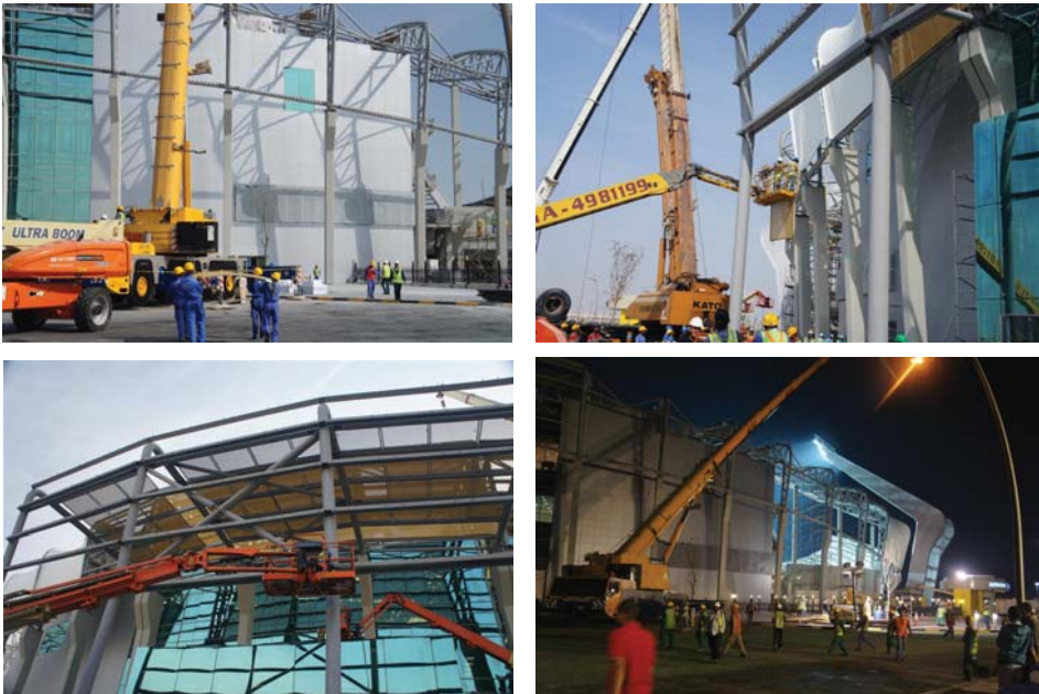
West Façade – installation
