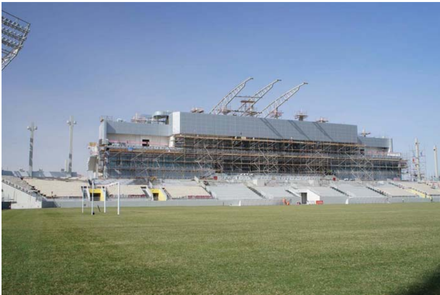
Steelwork installation on West Grandstand
