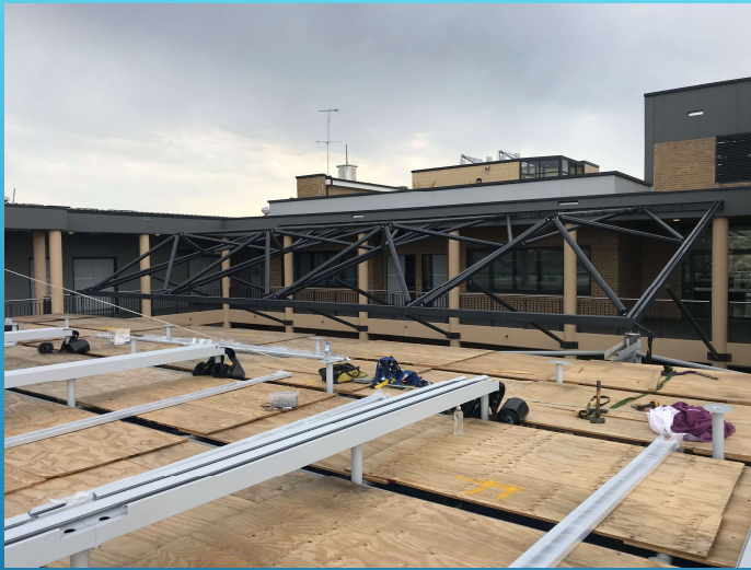
CONSTRUCTION OF THE LINK FRAME
