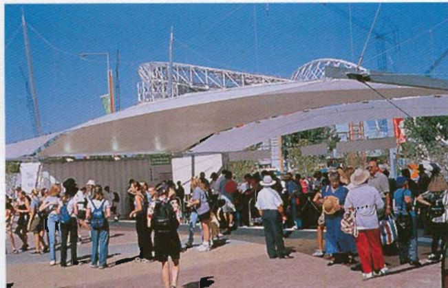
RAS - Temporary Entry Structure Shade Structures Pacific Pty Ltd
