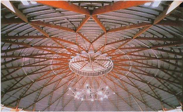
RAS Exhibition Halls Ove Arup & Partners Pty Ltd
