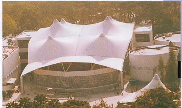
Ocean World Guangzhou Shade Structures Pacific Pty Ltd
