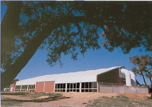
Waroona Aquatic Centre Höcker Structures Australia Pty Ltd
