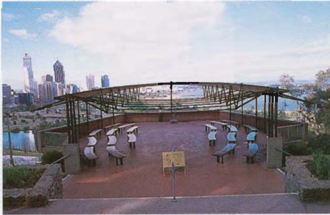
Kings Park Lookout - Temporary Fabric Structure Kenlow Pty Ltd
