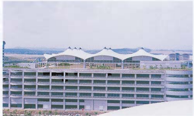
KL International Airport Carpark Roofs Permafab Pty Ltd
