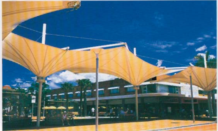
Entrant Shade Structures Birdair Specialist Consultant Shade Structures Birdair Project High Street Re-Development, High Street, Coffs Harbour, NSW Other Consultants Tract Consultants Architect Shade Structures Birdair Building Contractor Shade Structures Birdair Structural Engineer Shade Structures Birdair Other Contractor Ryan Earthmoving Pty Ltd
