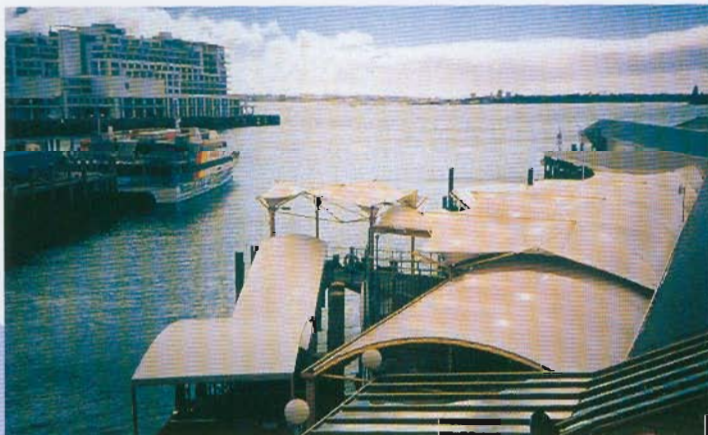
Entrant Structurflex Limited Structural Engineer Composolt Engineering Project Fullers Ferry Terminal Downtown, Auckland, NZ Specialist Consultant Structurflex Limited Architect Salmond Reid Architects
