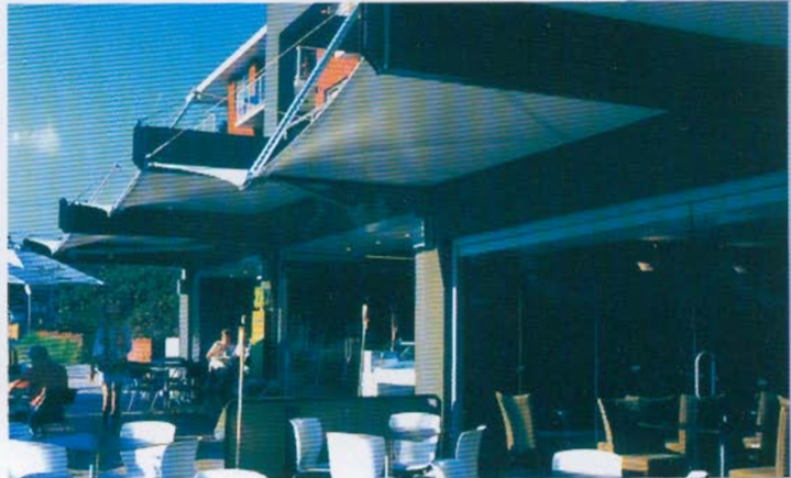
Entrant Shade Structures Birdair Structural Engineer Shade Structures Birdair Project The Strand Awning, The Strand, Dee Why, Sydney, NSW Specialist Consultant Shade Structures Birdair Architect Squillance Architects Building Contractor Shade Structures Birdair
